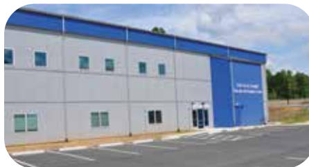
A-B Tech Entrance on right side of the building
